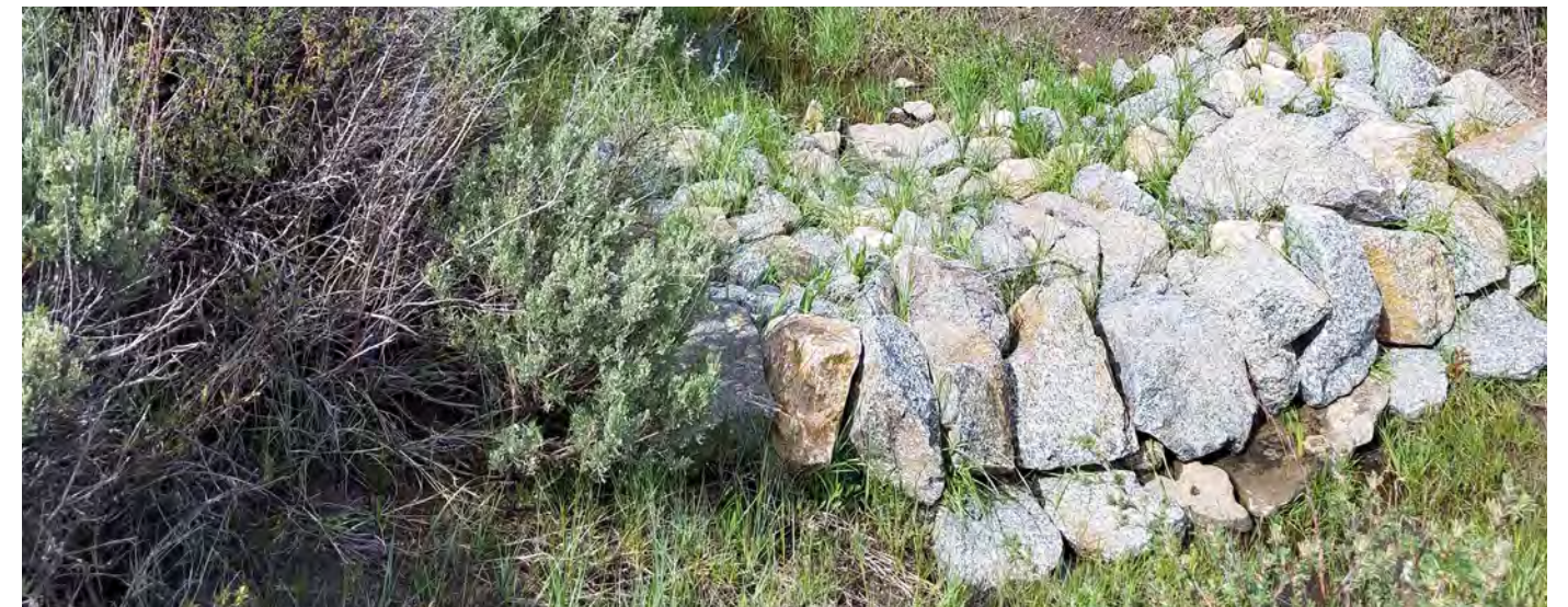
Upper Gunnison River Basin, Colorado, Zeedyk rock structures restoring an incised channel. Photo taken 2018 (credit: Nathan Seward, Colorado Parks and Wildlife).
