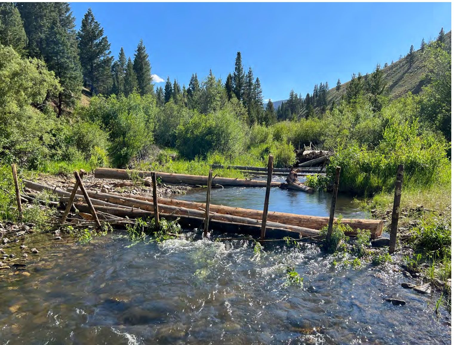
Panther Creek, example of Post-Assisted Log Structures (PALS). Photo taken July 15, 2022 (credit: Boyd Bouwes, Watershed Solutions, Inc.)
