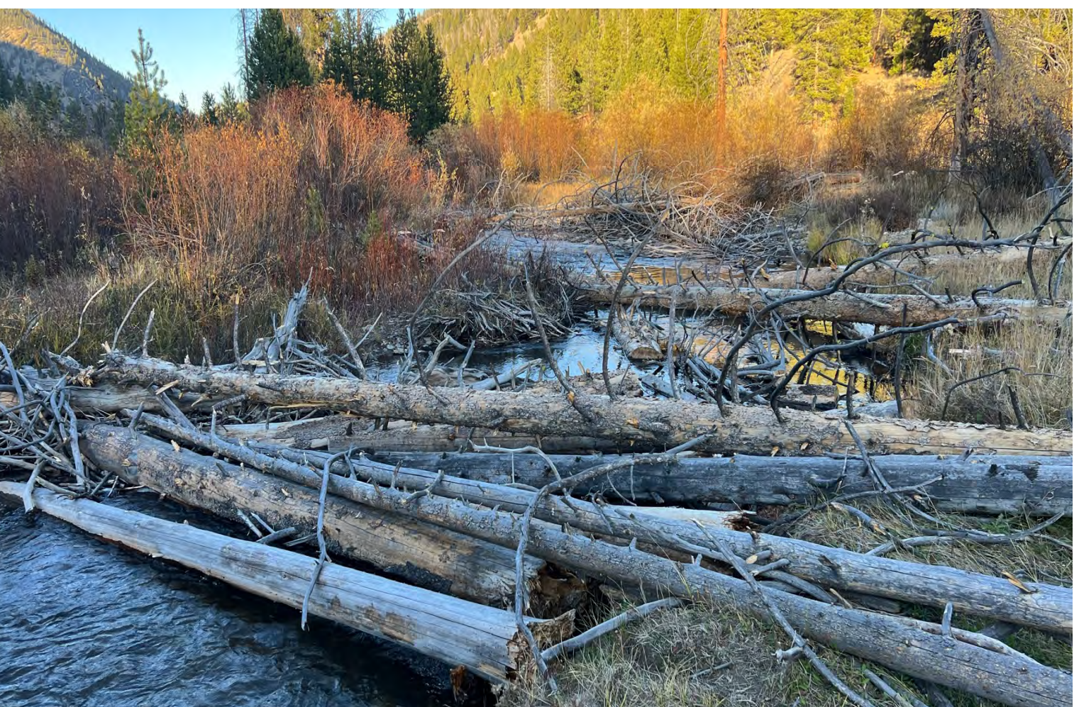
Panther Creek, example of an LWD addition. Photo taken July 15, 2022 (credit: Boyd Bouwes, Watershed Solutions, Inc.)
